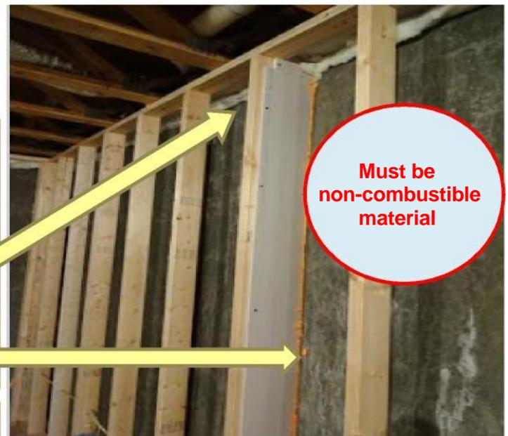
2. At all interconnections between concealed vertical and horizontal spaces such as occur at soffits, drop ceilings and cove ceilings.
