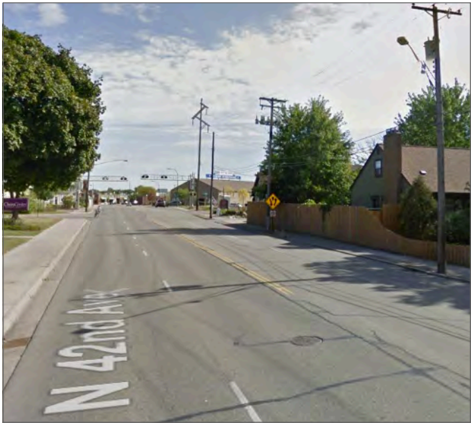
Existing conditions: Four 12' vehicle travel lanes. Image from Google Streetview.
