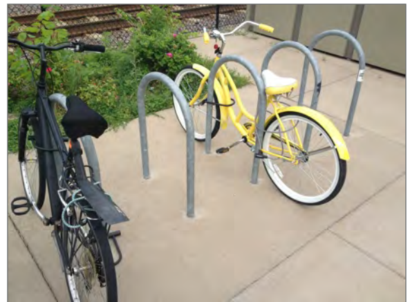
Inverted-U style bicycle parking should be installed at key destinations close to the primary entrance to the building.
