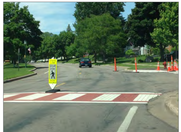
A shared-use path crossing of Shoreline Drive.
