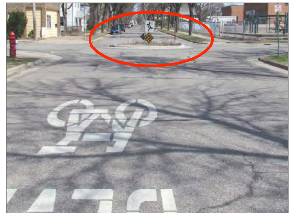
A neighborhood slow street in Northeast Minneapolis. A traffic circle calms traffic along this route.
