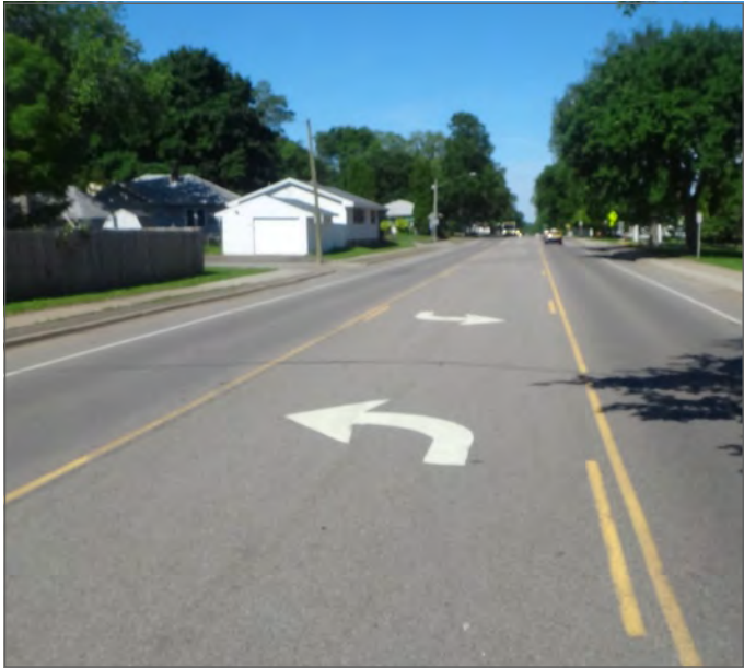
Existing conditions: Two 11' travel lanes and one 12' center turn lane with 5' paved shoulders.
