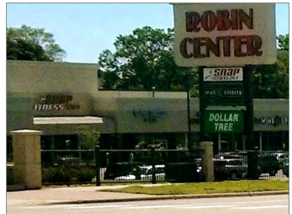
Navigating across parking lots to key destinations can be a challenge for pedestrians and bicyclists.
