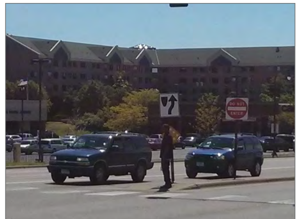
A pedestrian waits to cross Bottineau Boulevard at 41st Avenue N in Robbinsdale. This intersection has a high-visibility crosswalk, but would benefit from a “bull-nose” extension to protect pedestrians at the median, as illustrated below.
