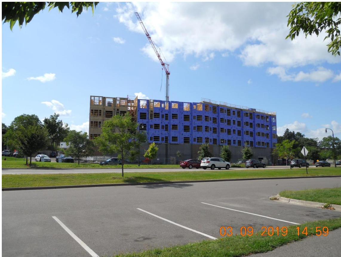
Figure 10: Birdtown Flats Apartments Under Construction
