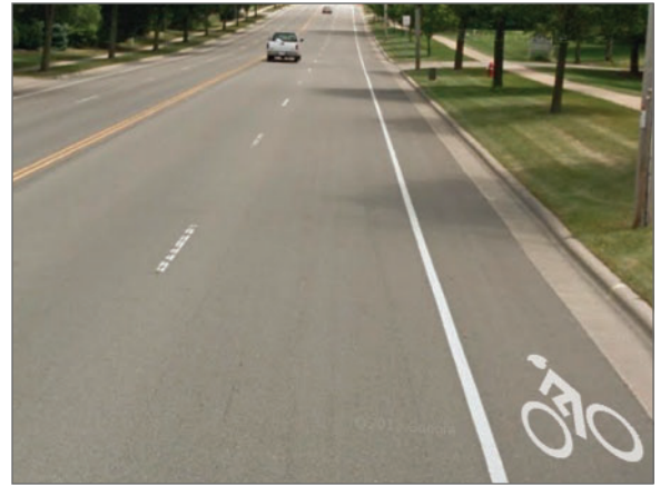
On-street bicycle lane created using the paved shoulder.
