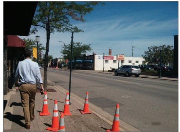
Maintenance work on a sidewalk in Downtown Robbinsdale.
