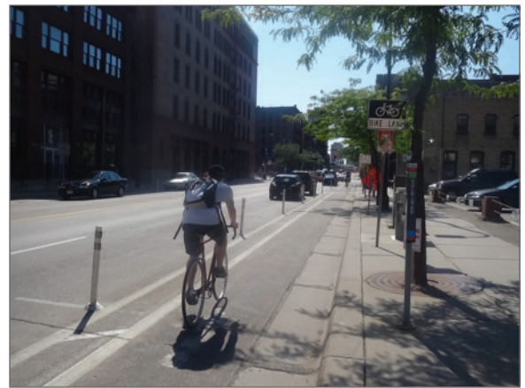
Cycletracks are a type of on-road bicycle facility that offer separation between bicyclists and motor vehicle traffic.
