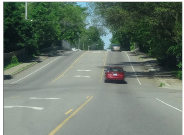
Travel lanes, a center turn lane, and paved shoulders on 36th Avenue N.
