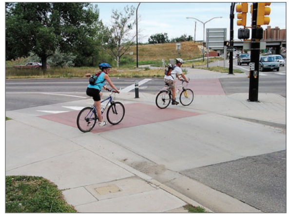
Raised and colored crosswalks slow right-turning vehicles. Courtesy of flickr, Richard Drdul.
