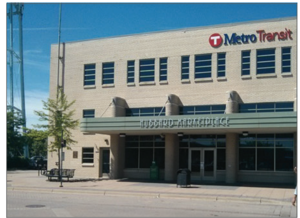
Hubbard Marketplace, site of the current Robbinsdale Transit Center and the future Bottineau LRT station.
