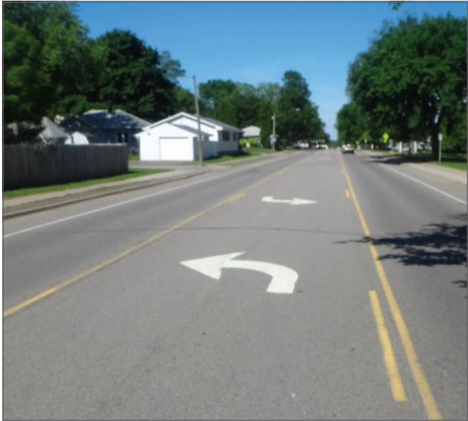
Existing conditions: Two 11' travel lanes and one 12' center turn lane with 5' paved shoulders.
