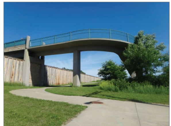
A pedestrian and bicycle bridge connects 39th Avenue North over U.S. Highway 100.
