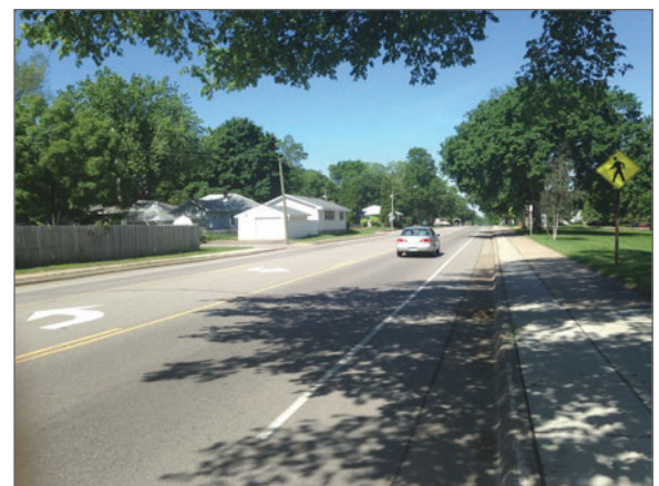
A paved shoulder facility on 36th Avenue North.
